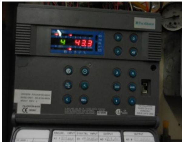
Liberty Elementary School – Boiler DDC Panel and Building Pneumatic Panel
