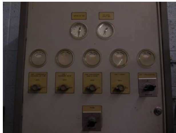
Liberty Elementary School – Boiler DDC Panel and Building Pneumatic Panel
