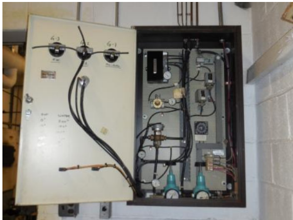
Central Elementary School – Pneumatic Panel and Time Clock
