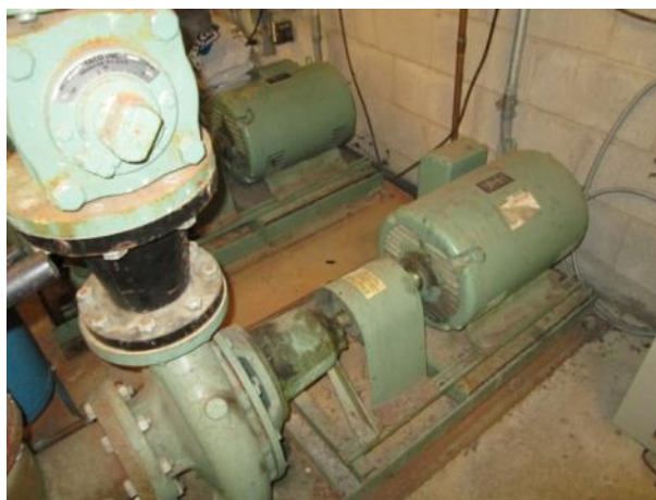
Great Meadows MS – WSHP Pumps and non functional VFD
