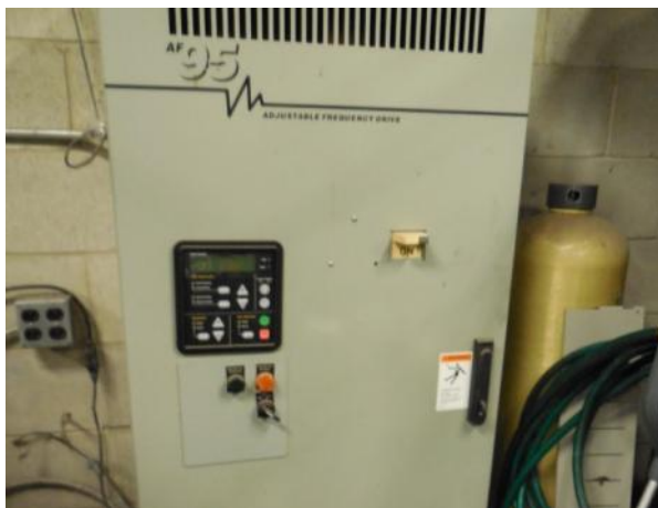
Great Meadows MS – WSHP Pumps and non functional VFD
